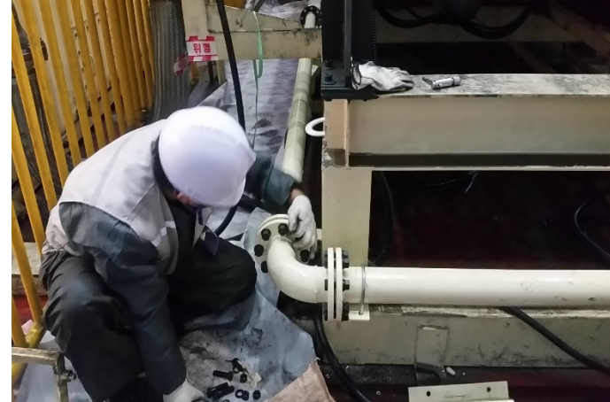
Washer Pipe Connection
